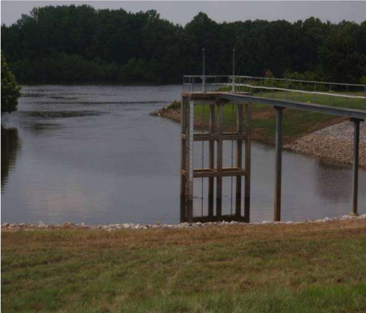
Lake Louis drawdown structure
